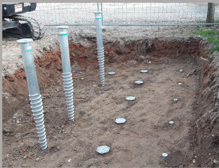
Fig. 1. View of the test screw micropiles
