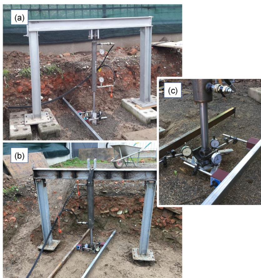
Fig. 5. Configuration of the tensile (a) and compressive (b) load tests, and measurement of pile displacement (c)
